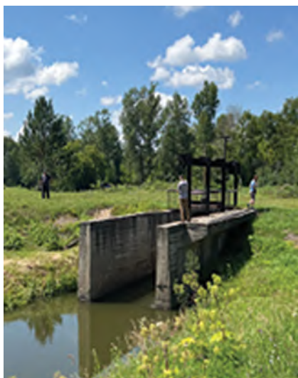
Fig. 2. The inlet canal of the water intake of the Losikhinskaya irrigation system:
